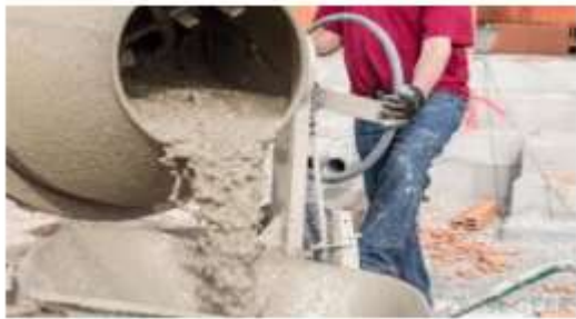
A VIEW SHOWING THE WET MIXING OF CONCRETE PLATE – 2 MIXING OF CONCRETE
